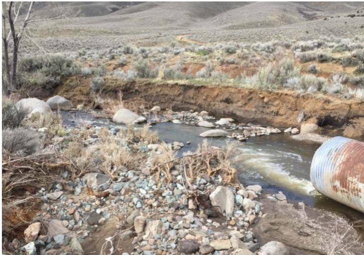
*(L) Downstream damage to creek from washed out culvert*
